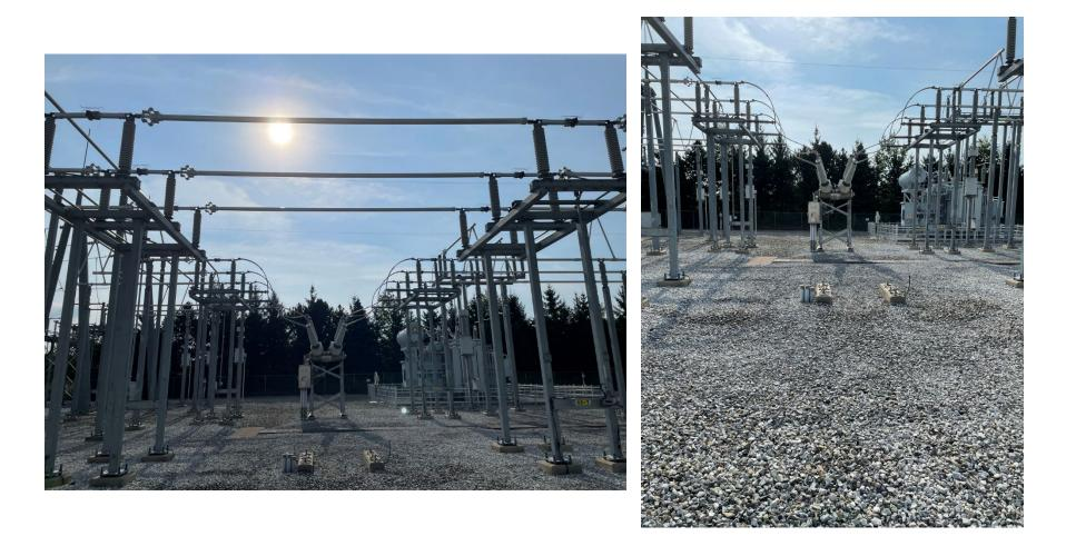
The future breaker position foundations and conduits are installed
