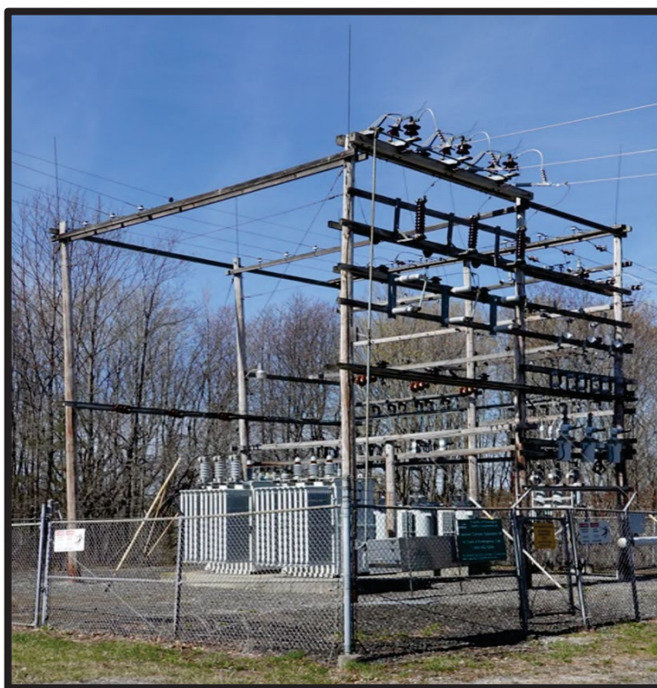
Figure 14: #8 Jackson Corners Substation – Wood Structure – 1968
