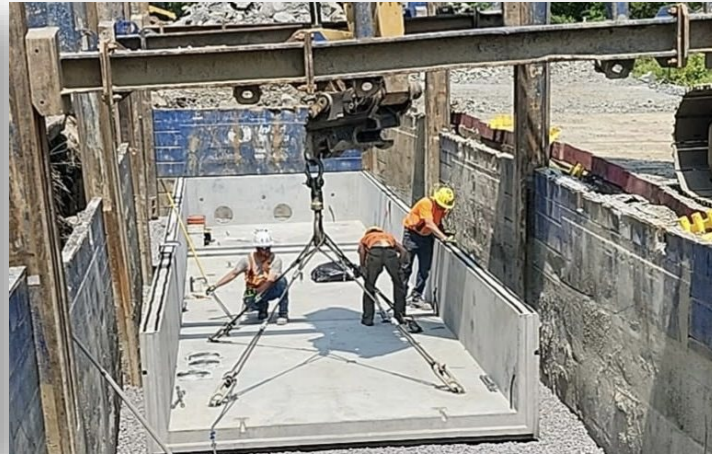
Splice Vault Installation
