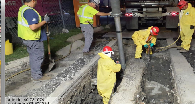
Night Hand Excavation
