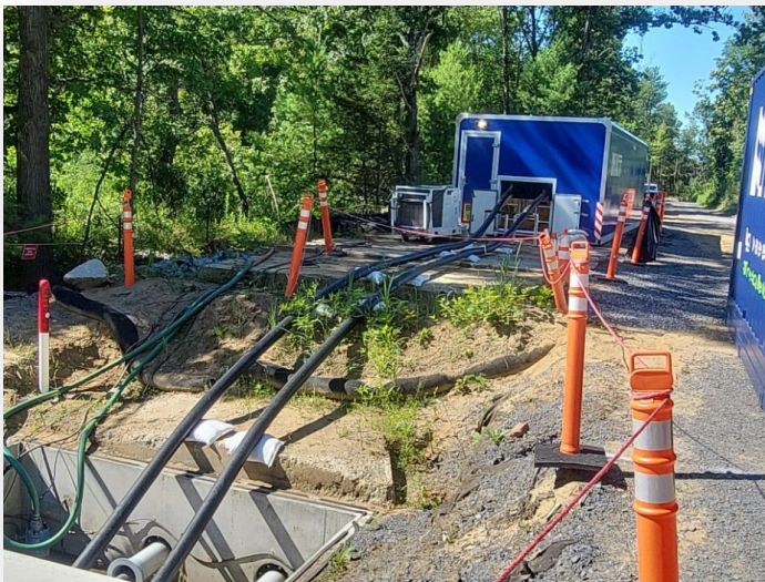
Hi-Pot Test Preparation
