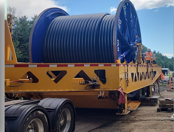
HVDC Wire Pulling
